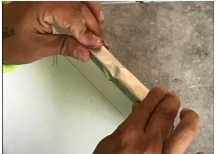
QuietRF® Shielding Tape application over QuietSeam® RF
