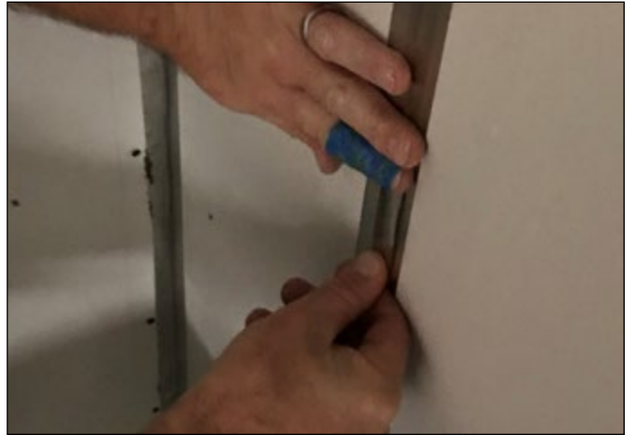
Applying QuietRF® Shielding Tape to seam
