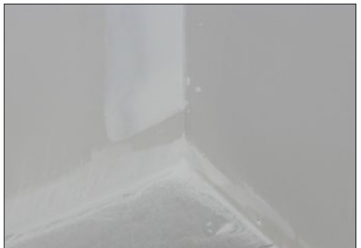
Finished QuietRock® 530RF at corner and floor
