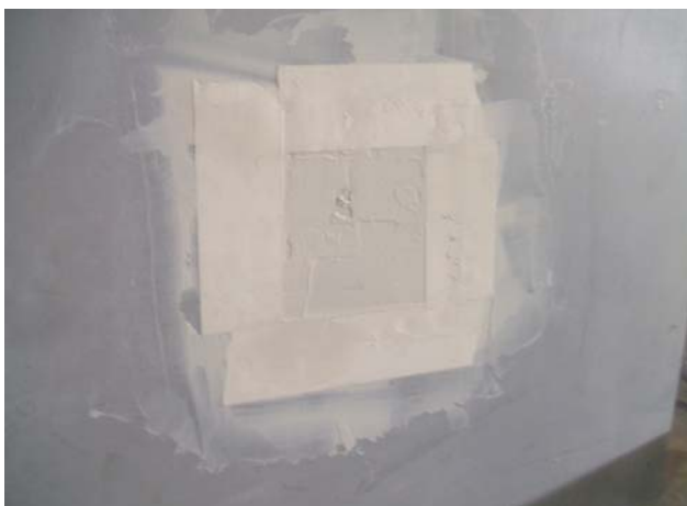
Figure 5: Tape and Finish Patched Area
