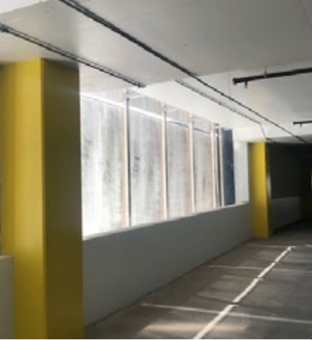
Metal screens on the inside of the parking garage
