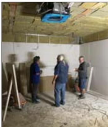
Full Exposure: QuietRock 545 installation over steel framing
