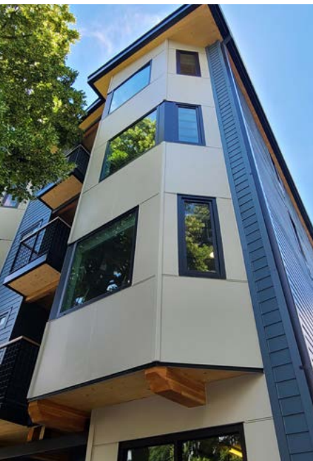
Exposed timber and blue cladding of the five-story, 17,000 square foot Chiles House building.
